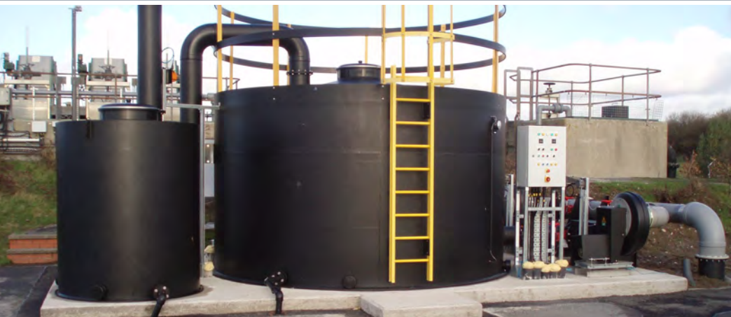
▲ Bio-trickling filter with polishing carbon filter for Dwr Cymru
