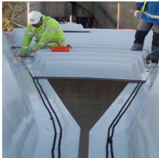
▼ Double seal arrangements and bolts fixed into embedded nuts within the GRP
