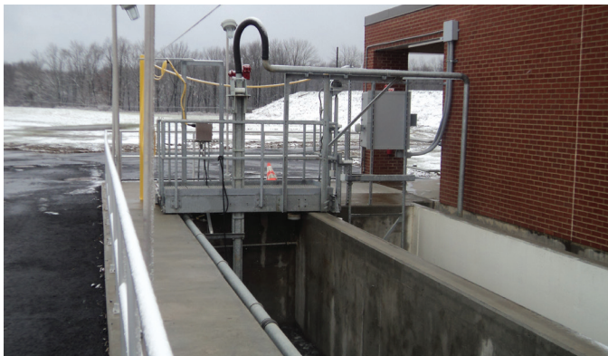
Bridges can be fitted with scrapers and/or pumps for grit removal.
